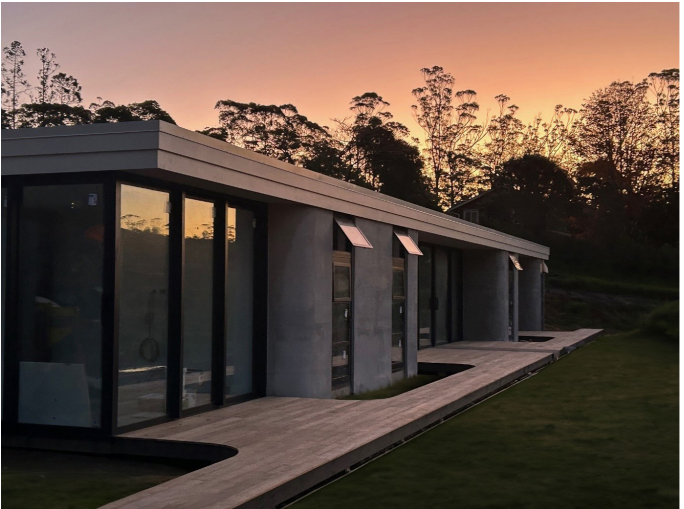
3D printed house in Pāremoremo, Auckland. Source: https://qorox.co.nz/news-and-media/first-fully-3d-printed-home-completed-in-paremoremo/
