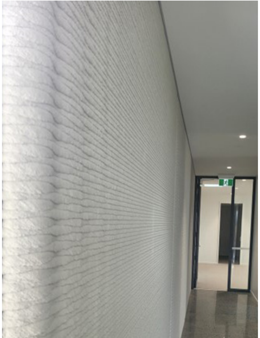
3D printed wall by QOROX. Source: https://qorox.co.nz/meeting-factory/
