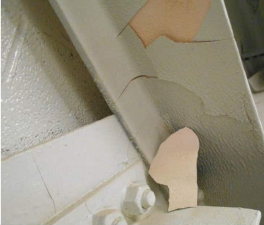
Damaged coating
